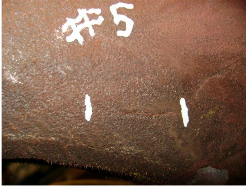
Figure D.30. Indication 5 (after 2 million cycles)
