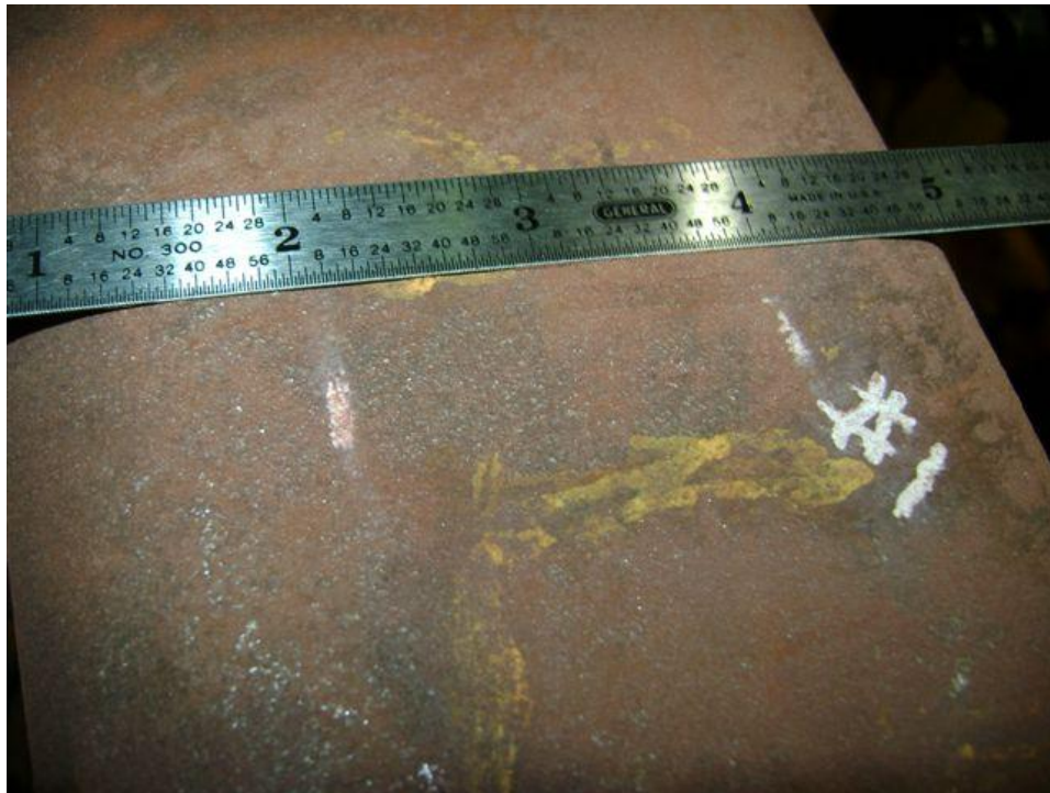
Figure D.31. Indication 1 at gage 8 (top of pedestal after 4 million cycles)
